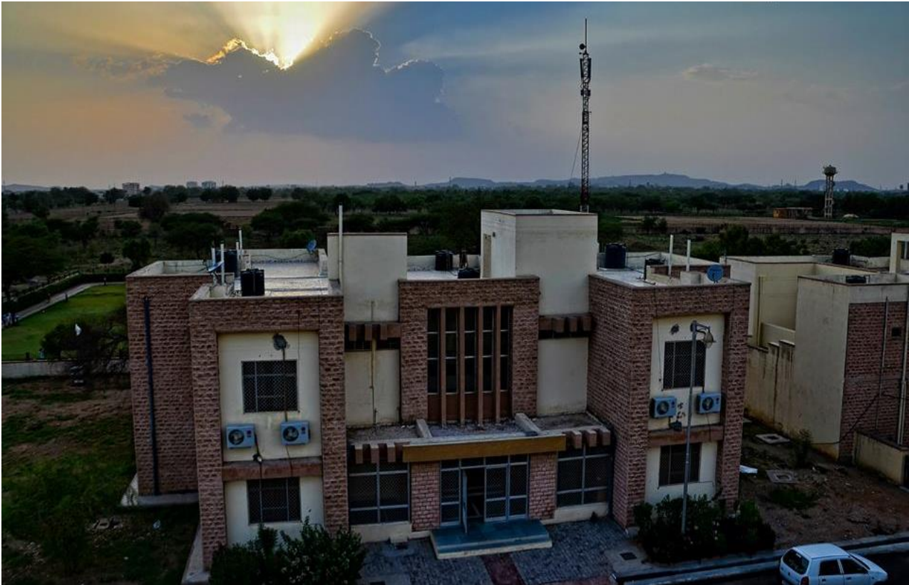
View of the Guest House
